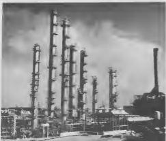
Fractionated in the NFAR towers, the LPG is stored in two tanks... Fraccioná den torenan di NFAR, e LPG ta ser warda den dos tanki...
